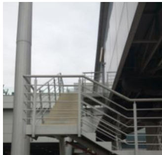
Example of escape route to be kept clear of FOD
