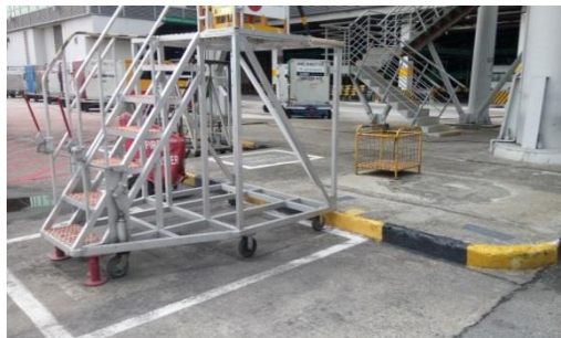
Example of plinth area to be kept clean of FOD and equipment returned to their designated position
